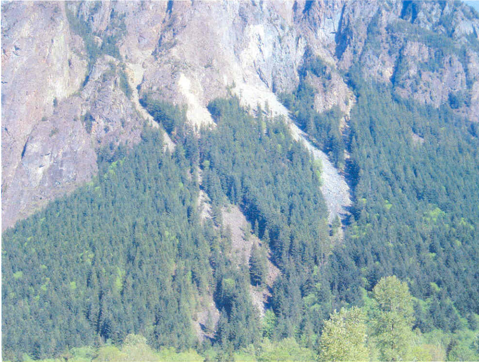
Photo 14: Rockfall from cliffs on the west face of Mt. Si has created the taluses seen here. Note areas of lighter gray on the cliff, suggesting active spalling of the cliff face.
